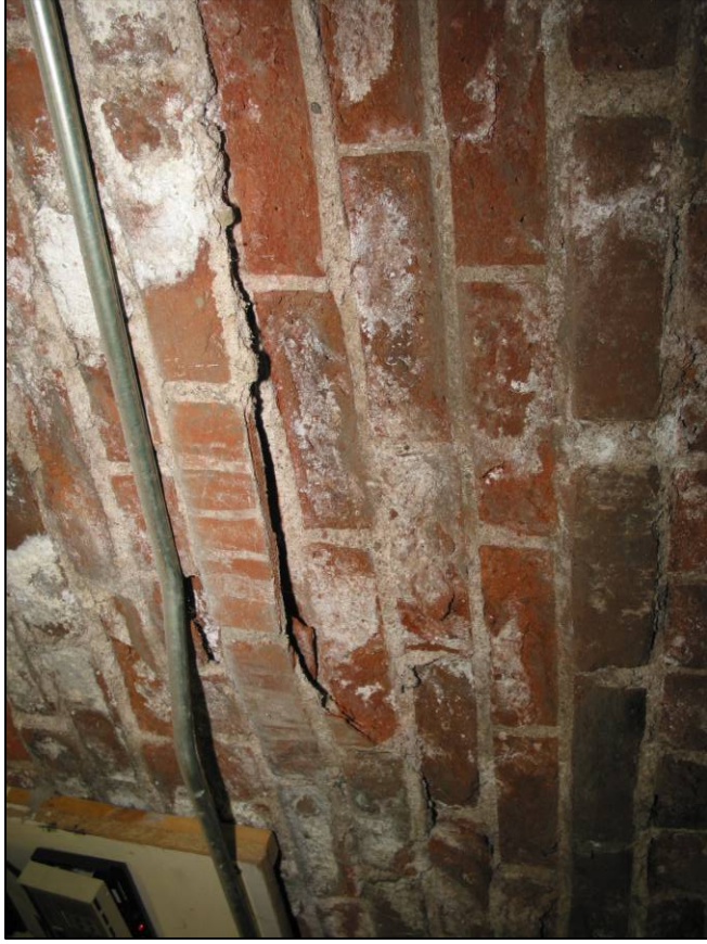
Efflorescence, a white chalky surface residue, indicates the presence of moisture and can cause significant deterioration of masonry.
