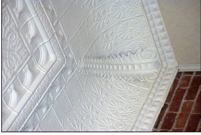
Tin ceilings should be checked for corrosion, staining, and other damage.
