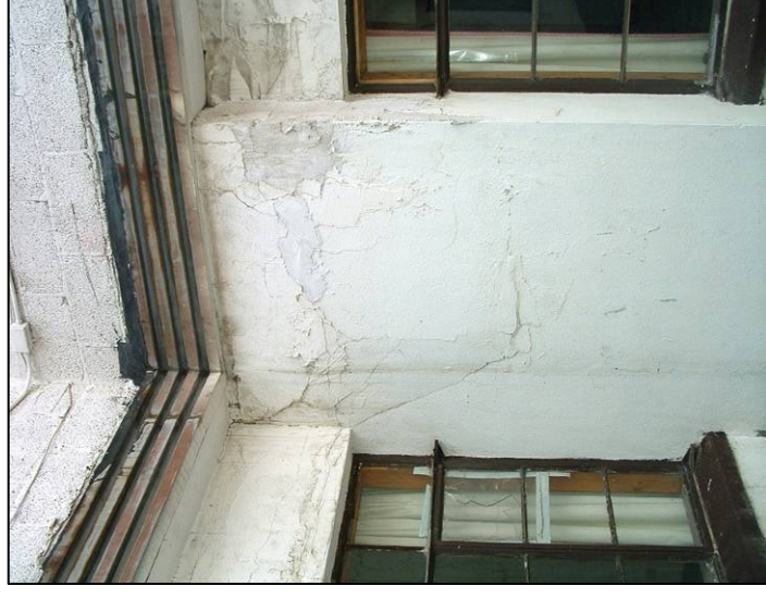
Cracks in stucco should be repaired to avoid moisture entering and enlarging them.
