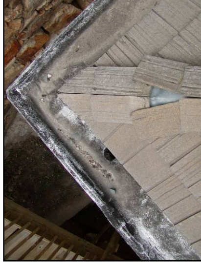
Missing or damaged shingles should be replaced as soon as possible.
