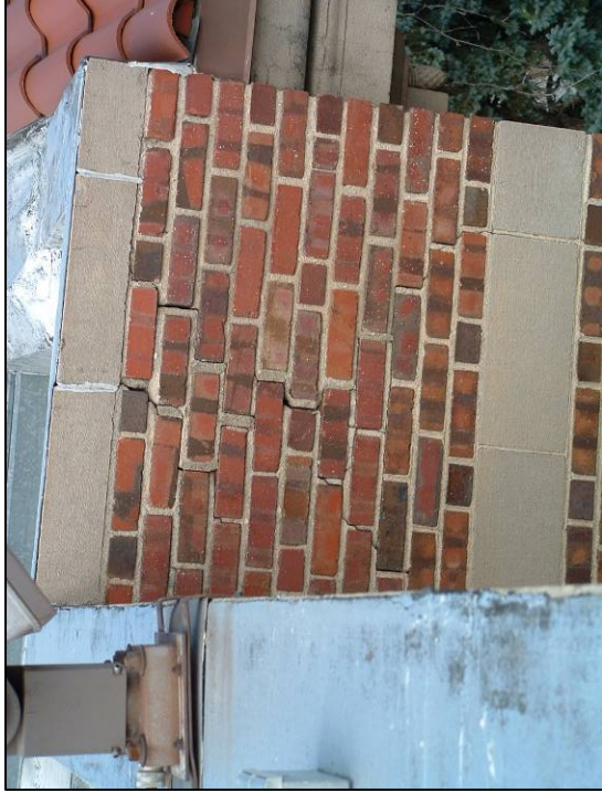
Masonry parapet walls are prone to moisture damage, such as deteriorated mortar joints, and should be examined regularly.
