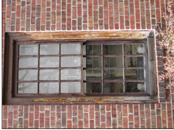
Lack of maintenance painting has caused this window to weather severely.
