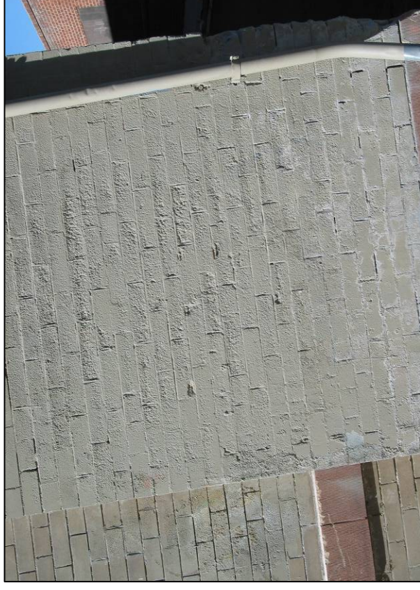
Destructive cleaning techniques such as sandblasting can damage masonry and other materials and should not be used.
